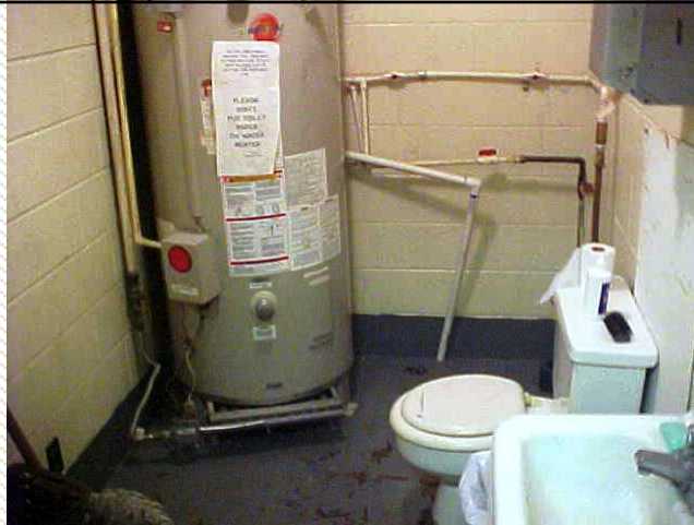
Gas fired water heater in a non-rated area
